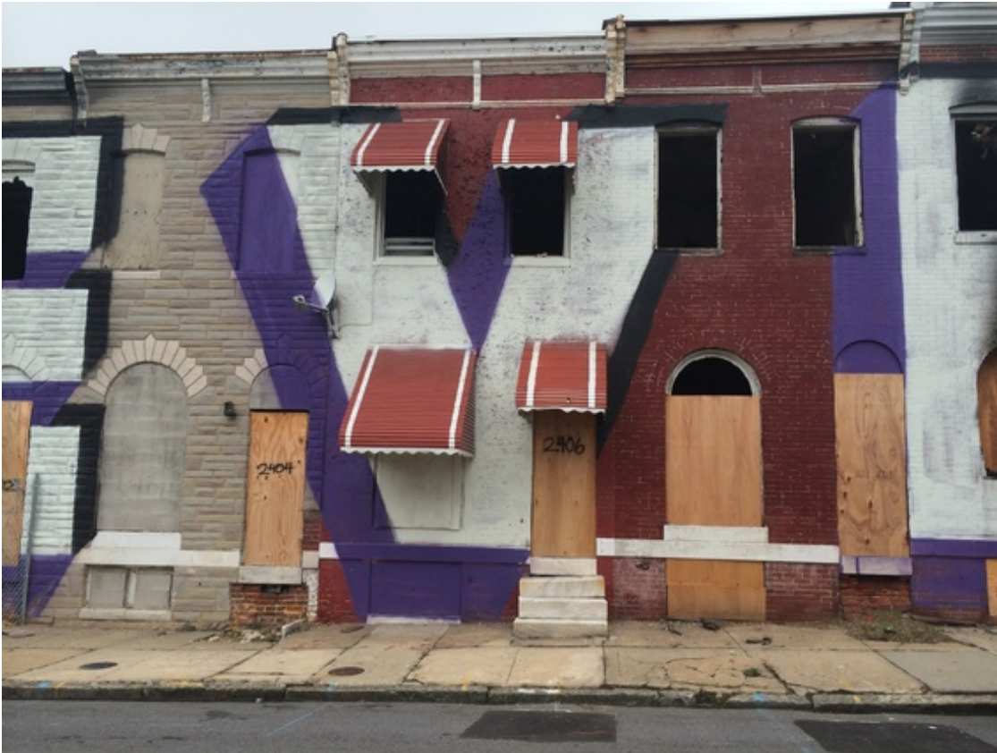
This row of vacants in East Baltimore is slated for demolition. (Alana Semuels)
